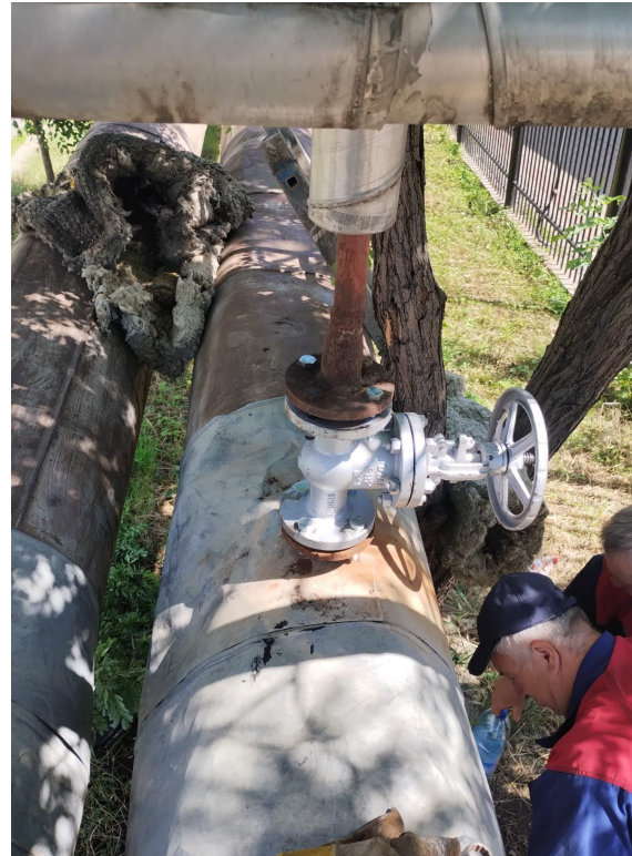
img 21, img 22 Rețea transport magistrala 3 vane Marimar
